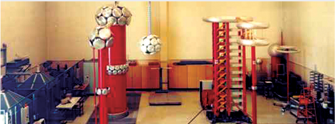
High Voltage laboratory
